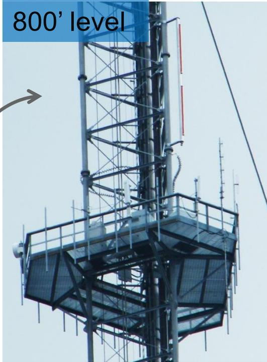
Base station antennas: Switchable between a vertically polarized and a circularly polarized antenna.
