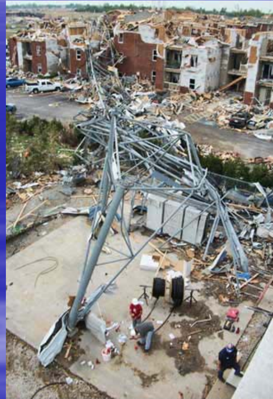
This 200-foot American Tower Corporation self supporting tower fell into a devastated complex that witnessed no fatalities after a tornado with wind speeds above 200 mph tore through Joplin.
