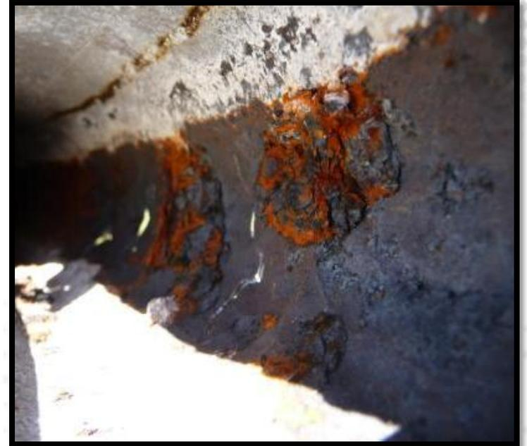
Galvanizing **NOT** Uniformly Deposited on Internal Portions of Pipe
