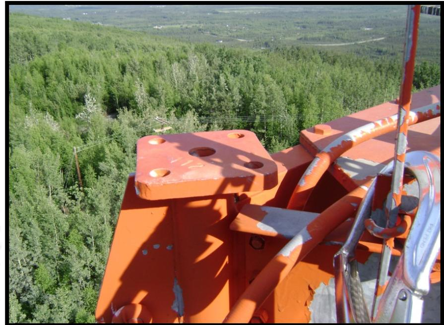
\*Pickling Acid Does Not Fully Drain Which Can Result in Poorly Coated Areas
