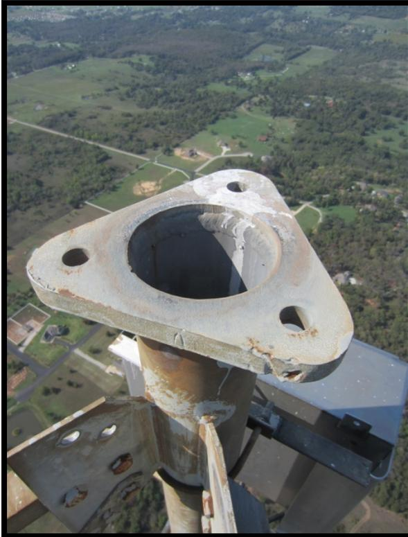
\*Butt Design ~ Poor Drainage
