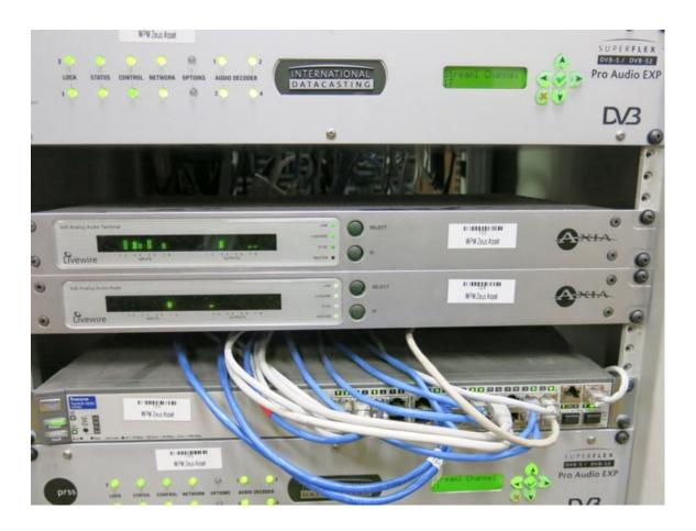
Satellite receivers integrate directly with system "Nodes" allow other audio sources to be integrated
