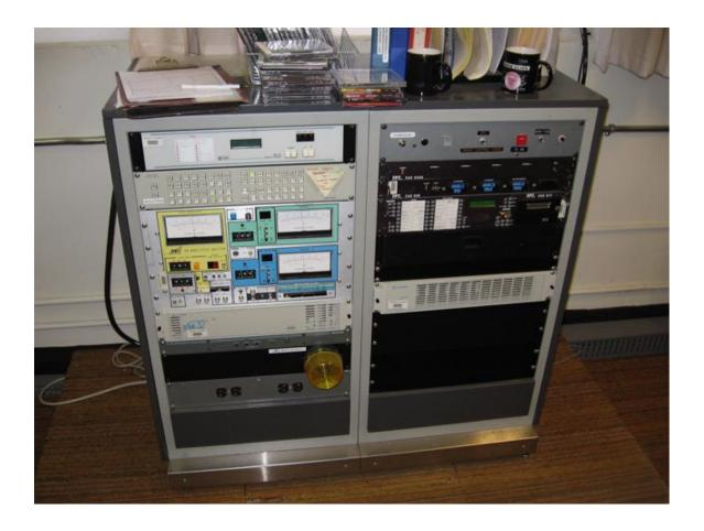
Leitch Via32 analog crosspoint router Leitch analog distribution amplifier chassis
