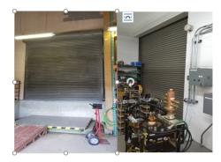
The current Harris/GatesAir Sigma transmitter, model CD3260P2, liquid-cooled transmitter is floor mounted to the left side of the site room and the GatesAir ULX-6300AT liquid-cooled backup transmitter system is floor mounted towards the center of the room. The new ULXTE-120 transmitter will be installed on the right side of the room in front of the dock doors.
