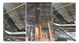
The distance for the RF transmission line for the input to the antenna switch is going to be about 60-feet. The RF transmission line output of the transmitter system travels to the RF combiners and into the transmitter RF waveguide switch. The run is about 10-feet. There needs to approximately 80-feet of RF line that will be needed for all the turns and bends to make it to the destination with 5 elbows needed to make all turns.
